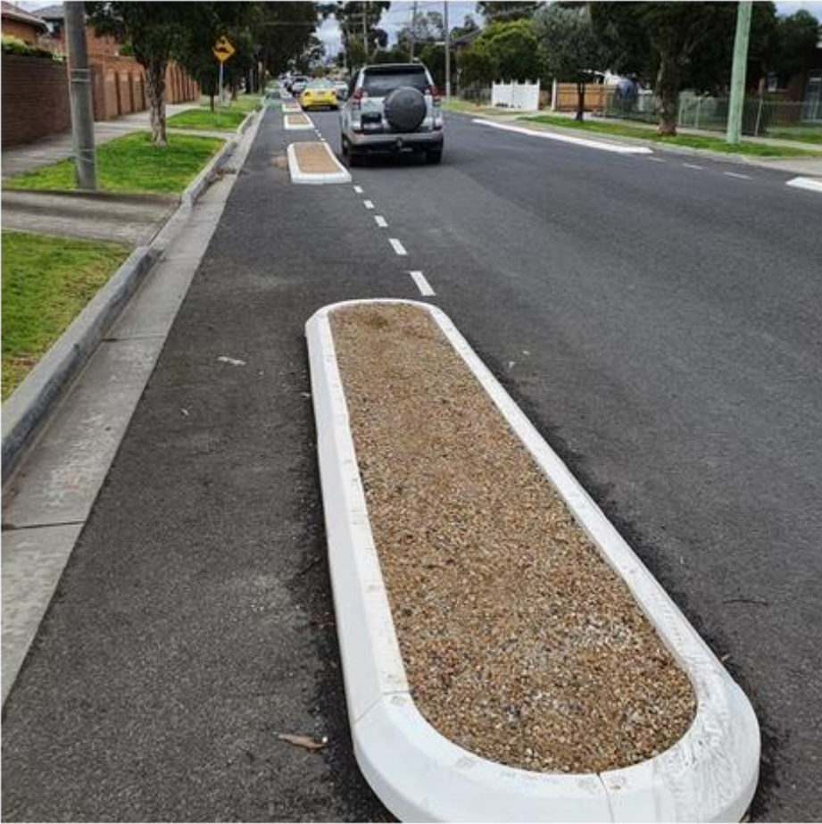
Example of traffic island used to separate cyclists from traffic and would suit separating pedestrians from traffic lane similar to a nature strip.
